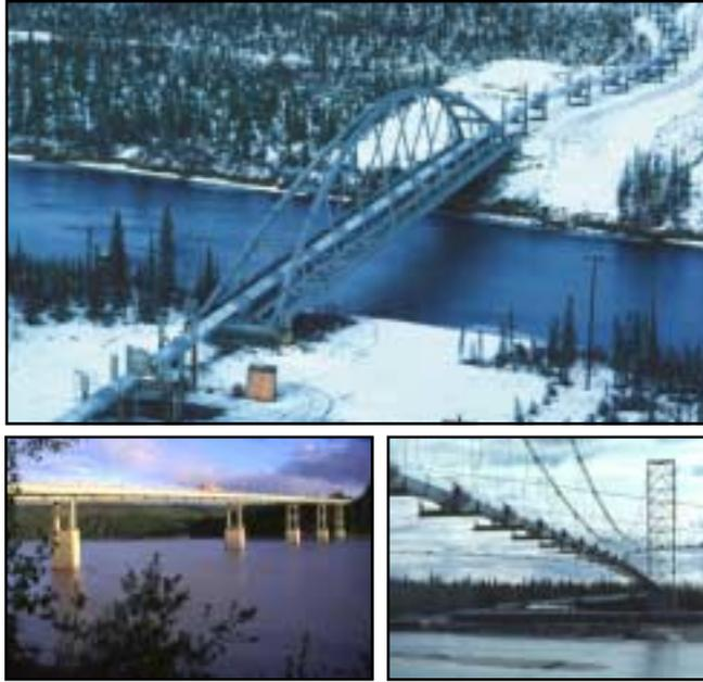
Photo 2.1-1. The above-ground pipeline is carried across the Gulkana River on a tied-arch bridge (top), the Yukon River on the same bridge as the Dalton Highway (bottom left), and the Tanana River on a suspension bridge (bottom right). (Alyeska photos)
