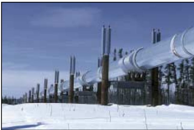
Photo 2-1. Vertical support members (VSMs) elevate the trans-Alaska pipeline in areas of thaw-unstable permafrost.
