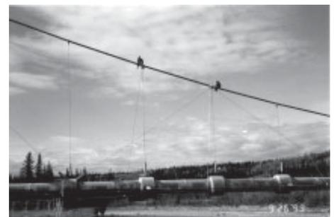
*These image show contractors inspecting the cables and fasteners on the Gulkana Bridge (JPO images by Lee Sires).*
